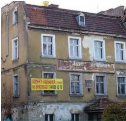
Old, pre-war building in Krzyżowa.
